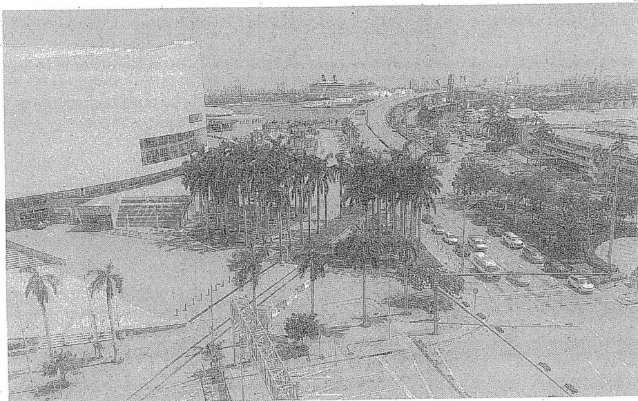
The area around the Freedom Tower where the author and her colleague found a man lying unresponsively on the sidewalk.
